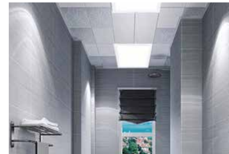
Ceiling Grid False Ceiling
